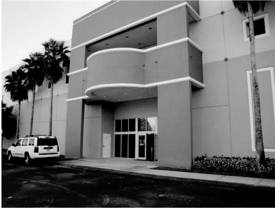
Figure 4-9 MDX AMTEC Facility
